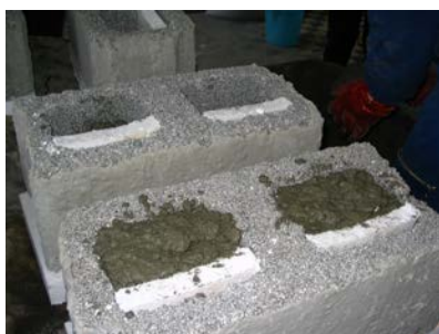
(a) Punjenje blokova svežim betonom Filling with fresh concrete
